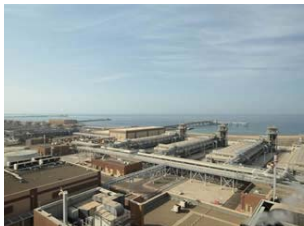
SWCC seawater desalination plant in Shoaiba, Saudi Arabia
