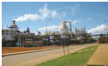
Bioethanol plant in Santa Juliana
