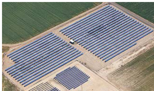
Solar power generation system constructed by Stellar Energy (a subsidiary of Soligent) at the world's largest winery (California, USA)
