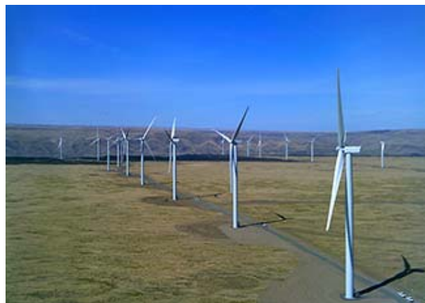
Shepherds Flat power plant
