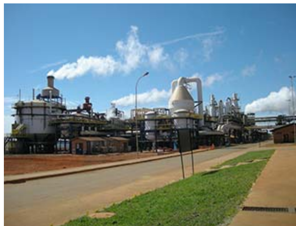
Bioethanol production plant in Santa Juliana
