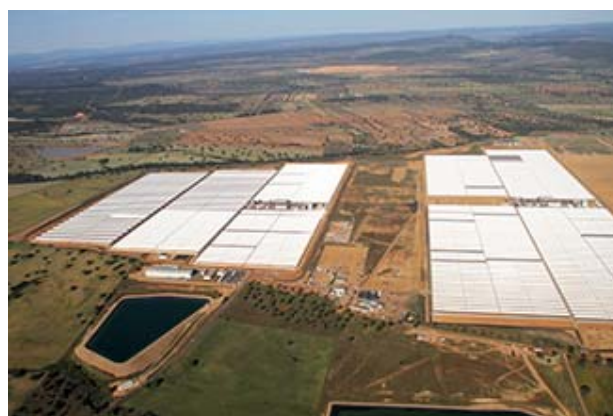
Two solar power plants jointly operated with Abengoa Solar
