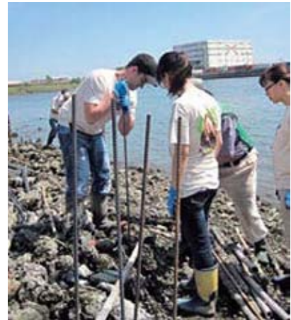
Assembling a bamboo tidal barrier
