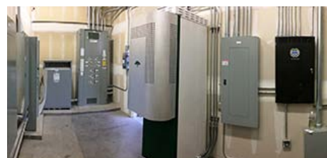
Green Charge Energy Storage
