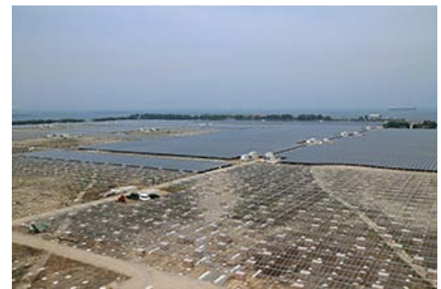
Steady progress of construction at the Oita Large-Scale Solar power plant
