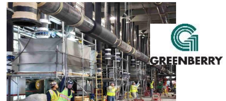
Piping Fabrication and Installation
