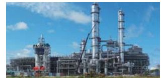
Methanol Plant in Brunei (Manufacture of methanol)
