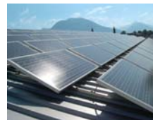
Procurement of solar panel parts
