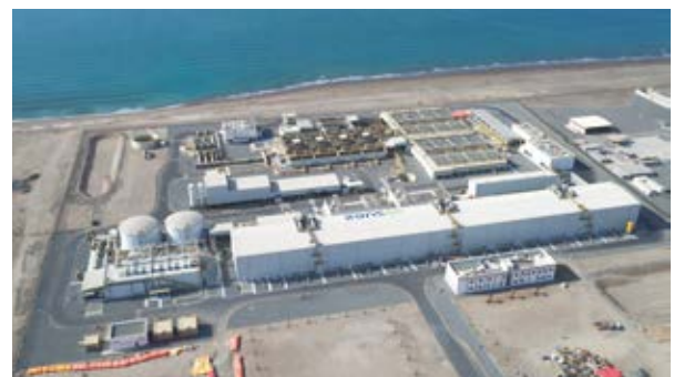
Barka Seawater Desalination Plant in Oman
