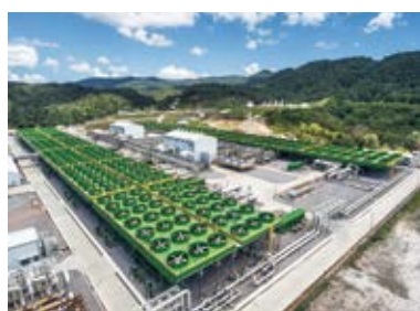
Sarulla Geothermal Power Plant, Indonesia
