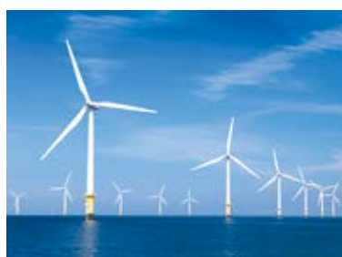
Butendiek Offshore Wind Power Plant, Germany
