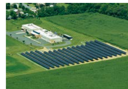
Nazareth Solar Power Facility in Pennsylvania, USA
