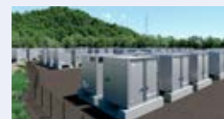
Large-scale energy storage facility under construction in Fukuoka
