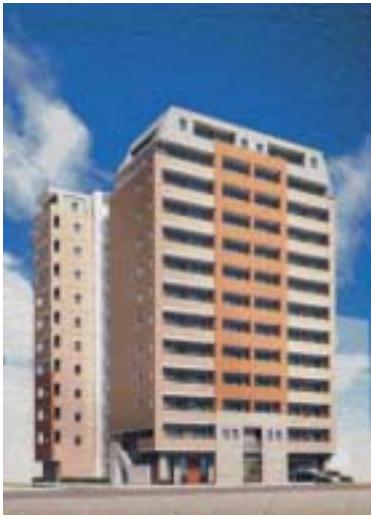
A condominium building in central Tokyo which is included in the private fund
