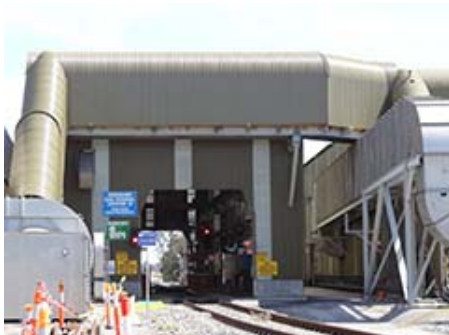
The rail receival station where coal is unloaded from coal trains onto conveyors.
