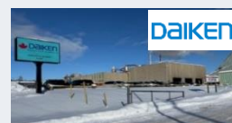
DAIKEN North America Manufacture of interior wood boards
