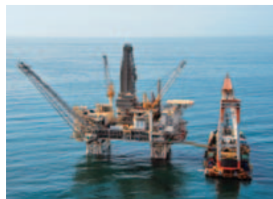
【写真提供】AIOC (Azerbaijan International Operating Company)
